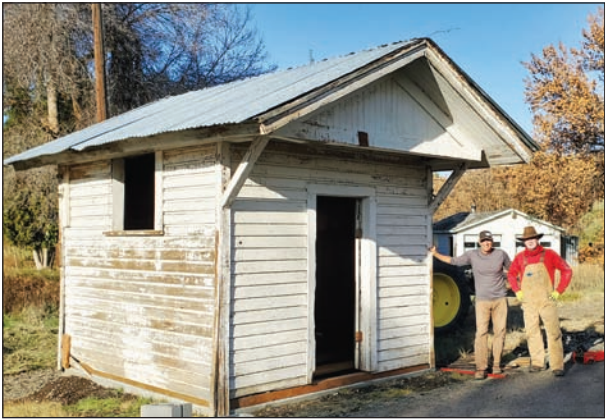
The old Eaton Train Depot will soon get a new roof, which has been needed for some time. Above is Ray Laan, left, and Kevin Jones. Photo courtesy of Weiser Architectural Preservation Committee
